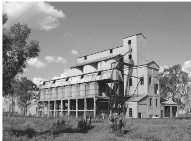
Grain elevator at Davel, South Africa. This disused grain elevator, built in 1924 for South African Railway, is one of an extant network of 33 country elevators provided in the maize-growing region to promote exports and the interests of farmers. PHOTOGRAPH BY DAVID WORTH, 2001
